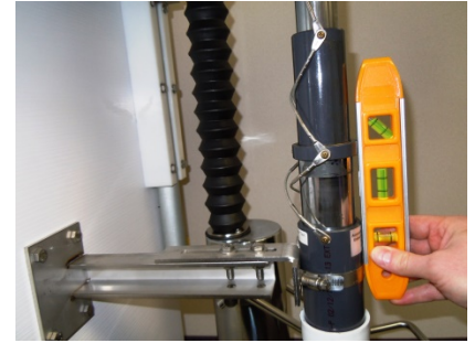
adjust bracket so drain is plumb
