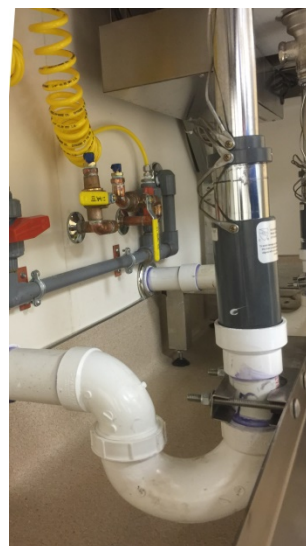
Drain mounted to sink frame cross member
