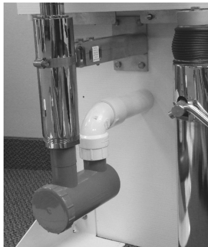
1701 Hair Trap typical installation
