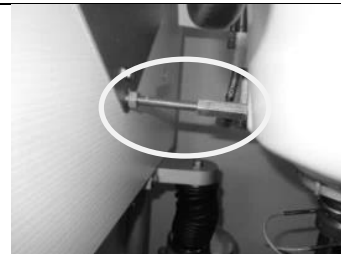
some sinks have leveling bolt
