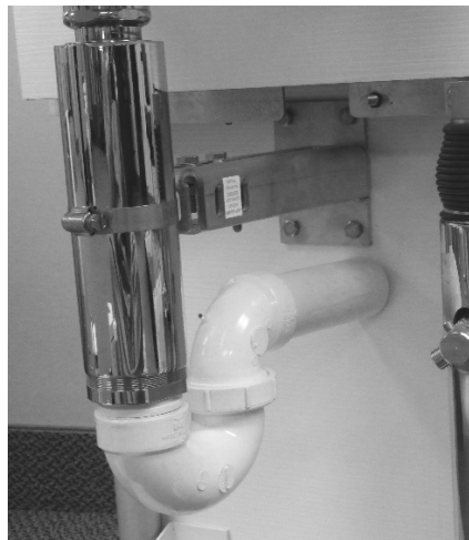
P-Trap typical installation
