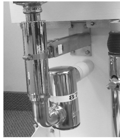
Cast Iron Hair Trap typical installation
