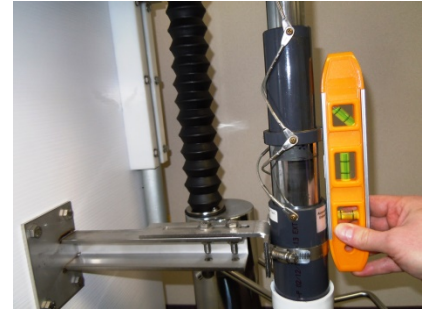
adjust bracket so drain is plumb
